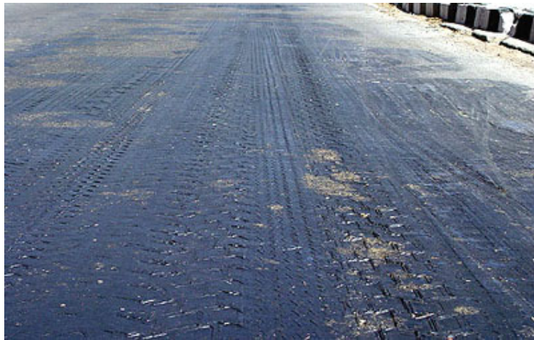
Photo: bitumen road (without plastics)
