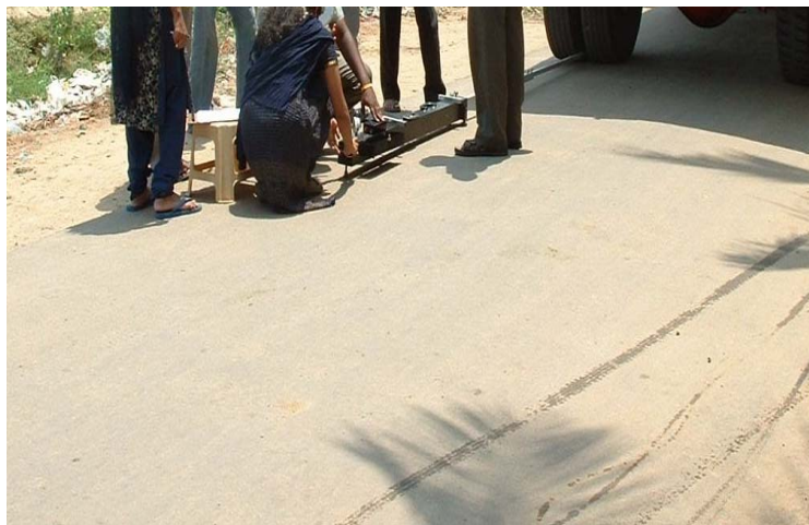
Photo : Vandiyur Main road
