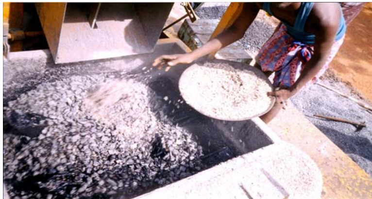
Photo: Mixing of Shredded Polymer on coarse aggregate
