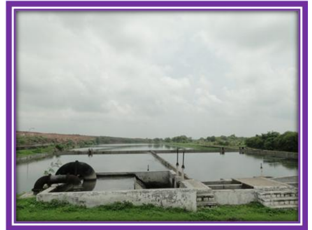
Anaerobic followed by facultative ponds
