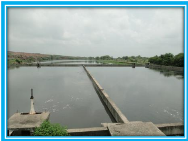
Anaerobic followed by facultative ponds
