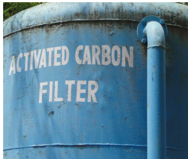
Activated carbon filter
