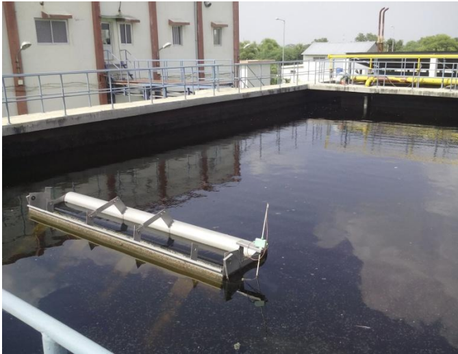
Processed Water Decanting
