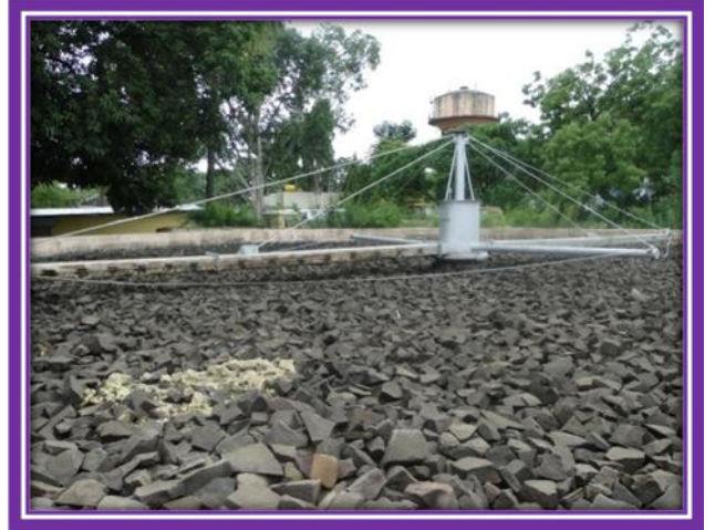
Trickling Filter
