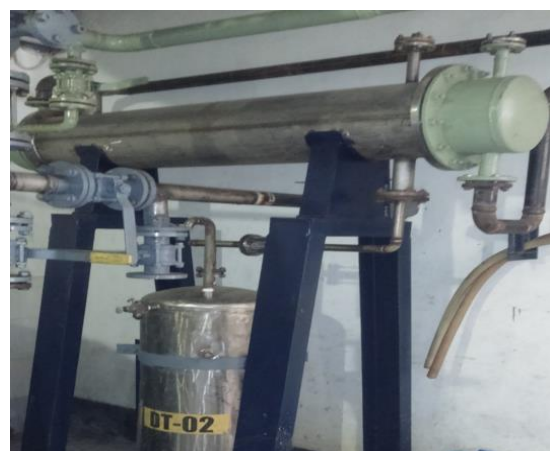
Figure 9: Solvent Vapour Recovery System
